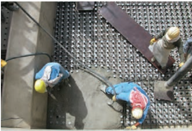
Pouring and vibration of concrete.
