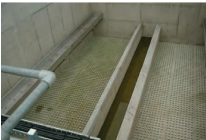
Finished filter floor with caps removed and filter nozzles installed.
