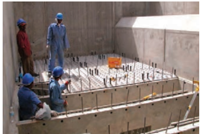
GRC panels being positioned on dwarf walls.
