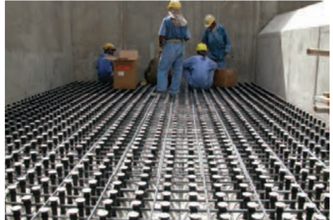
Installation of all threaded sleeves and protection caps.
