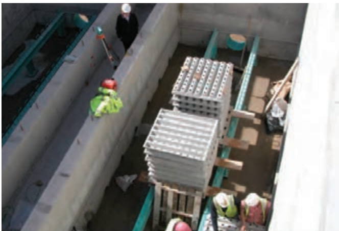
GRC panels being positioned on alternative steel support structure.
