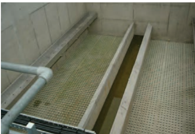
Finished filter floor with caps removed and filter nozzles installed.
