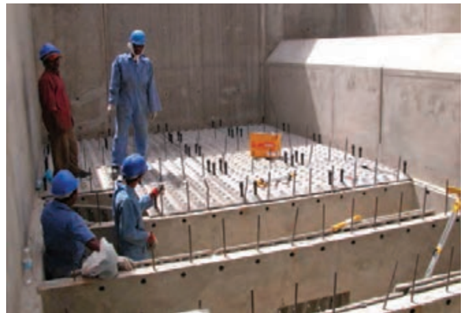
GRC panels being positioned on dwarf walls.
