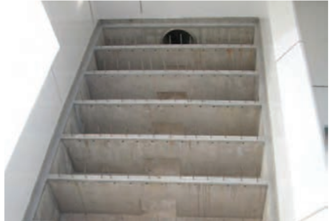
Civil support structure ready for filter floor installation.
