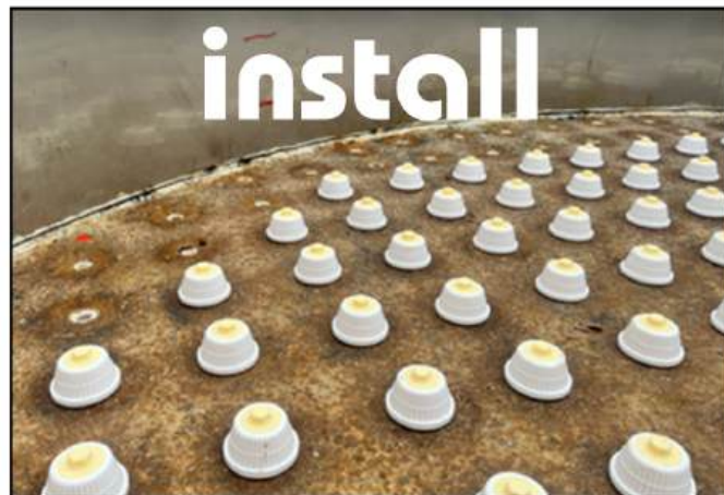
3. Clean filter, supply and install nozzles
