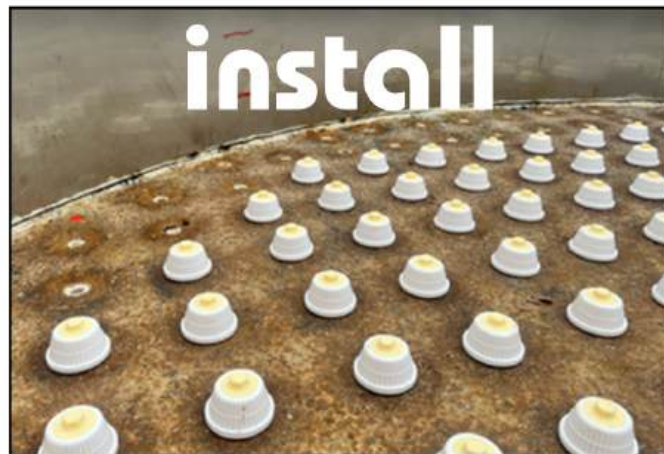
3. Clean filter, supply and install nozzles
